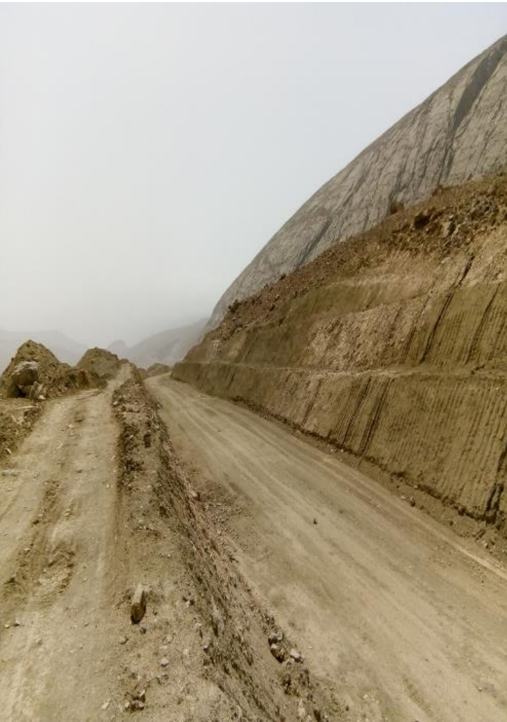
COMMON EXCAVATION OF ACCESS ROAD
